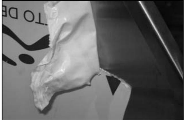
Remove any protective plastic prior to installation.
